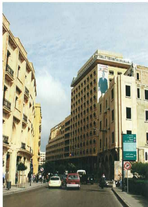
Azariyeh building, where JaCMES is situated, has long been a landmark of Downtown Beirut.
